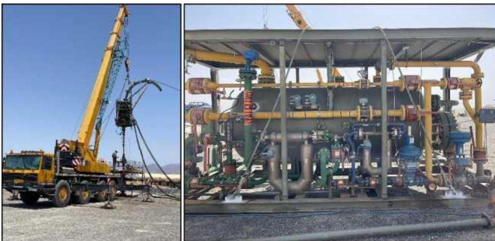
MOU-3 "A" Sand rigless testing - coiled tubing unit and nitrogen lift
